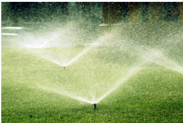
High Use Inefficient Fixed Spray Sprinklers
