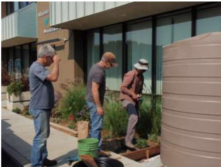
MPWMD staff installs a solid pad at the base of the Monterey cistern demonstration site
