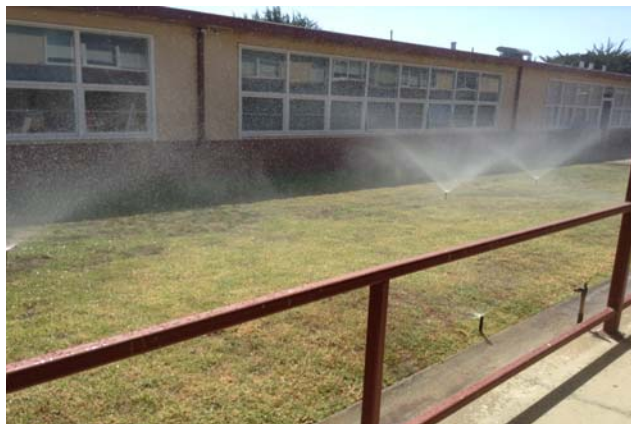
High Water-Use Inefficient Fixed Spray Sprinklers
