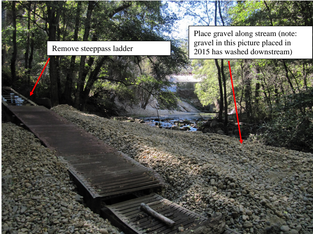
Figure 1 – Abandoned Alaskan steppass fish ladder downstream of Los Padres Dam
