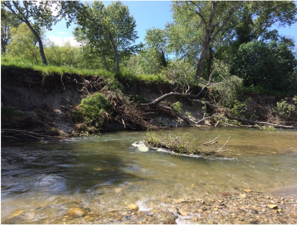
Figure 2. Left streambank after winter of 2017 erosion event (note lack of protective vegetation)
