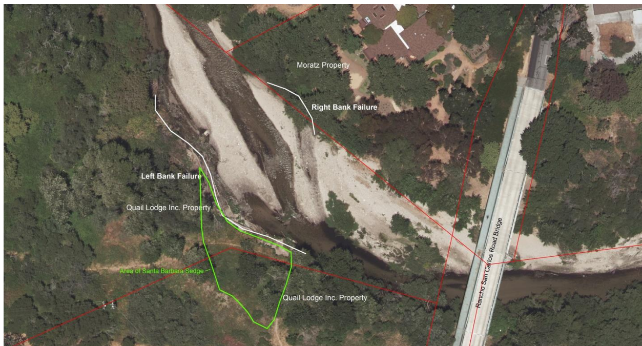
Figure 3. Aerial image showing locations of erosion just downstream of Rancho San Carlos Road Bridge
