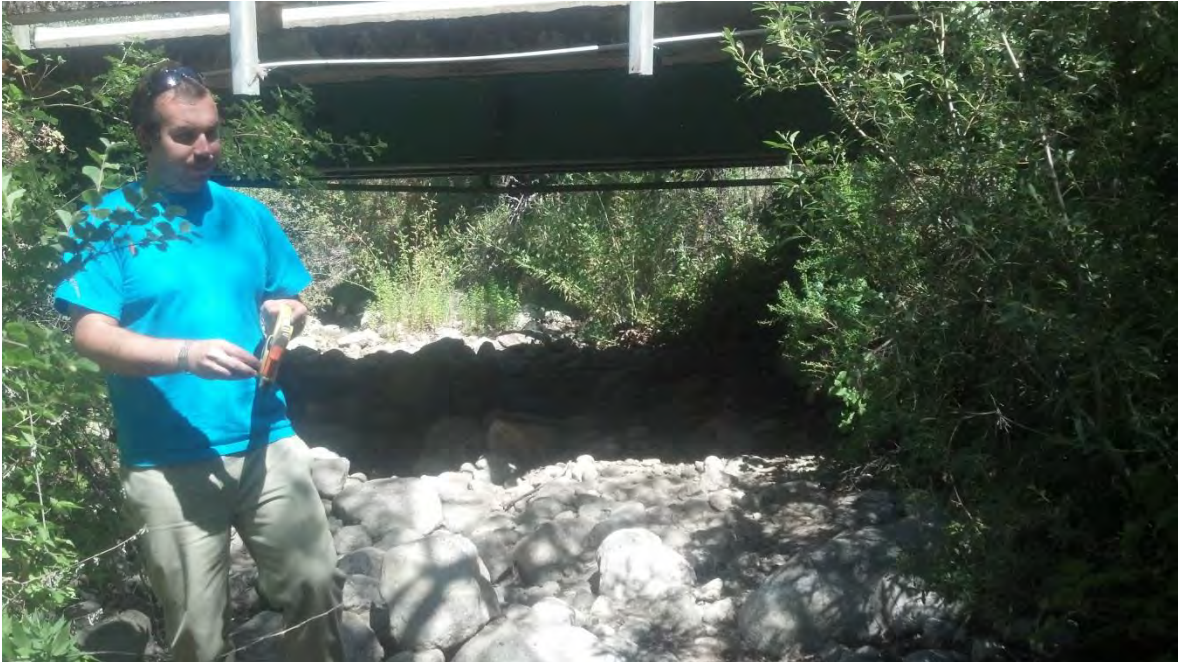
Site UCC-5. Looking upstream.
