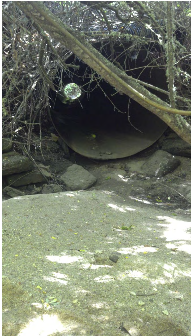
Site PCB-5. CVAC culvert outlet and plunge pool.
