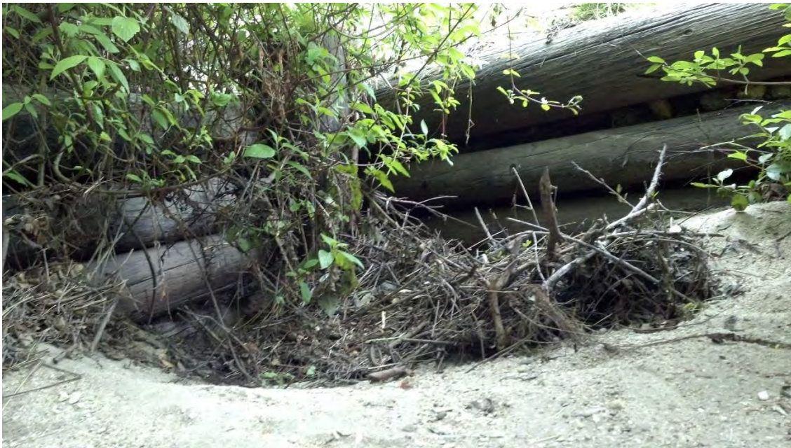
Site PCB-2d. V-notch log weir, looking u/s.
