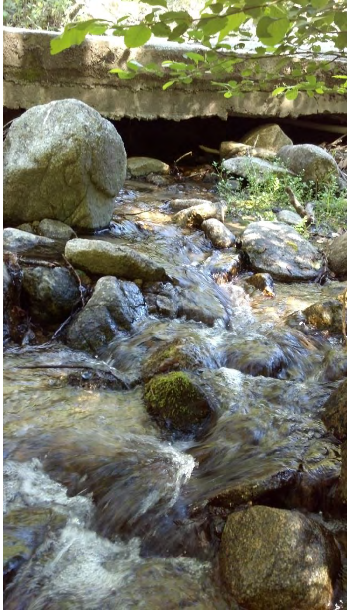
At low flow, the entire creek passes underneath the ford where passage is blocked by woody debris and rocks.
