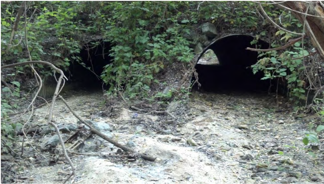
Site PCB-3. Valley Greens Rd. culverts - Looking upstream.
