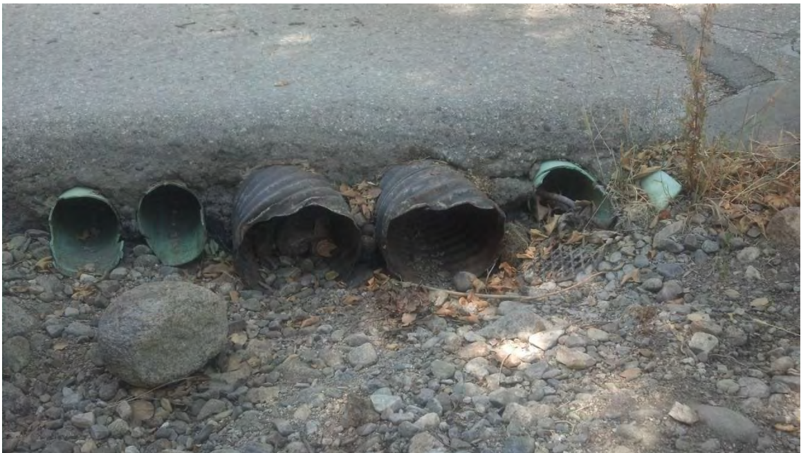
Site UCC-3. Close-up of the culvert inlets.
