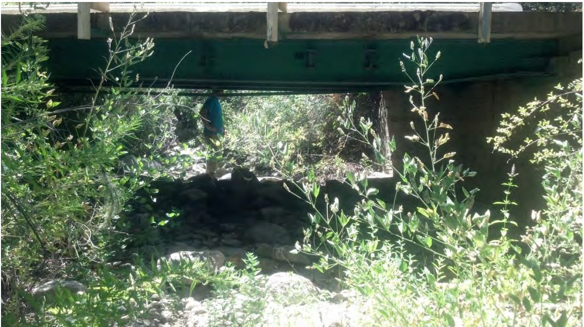
Site UCC-5. Looking downstream.
