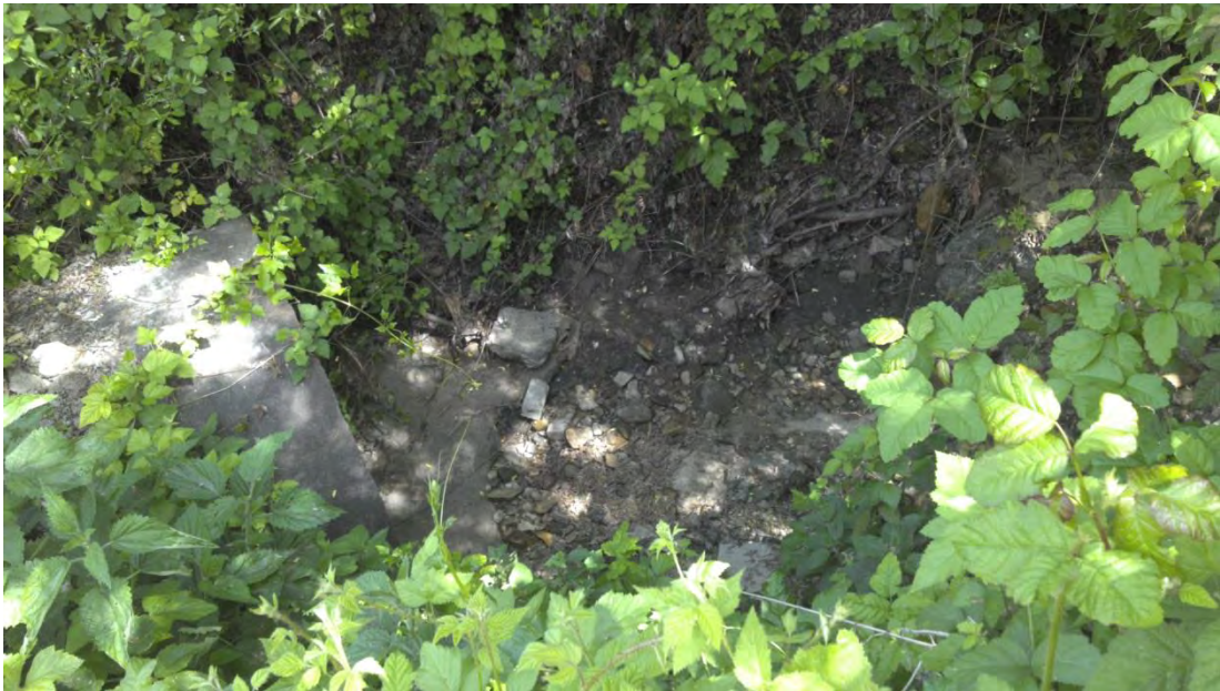
Site PCB-5. Inlet and channel u/s of culvert.
