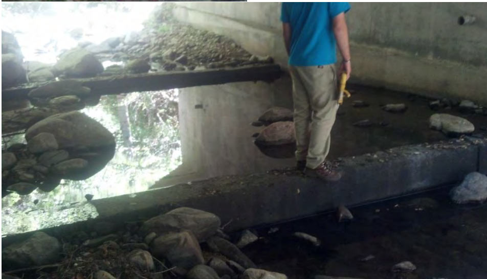
Site UCC-9. Looking upstream, and close-up of the concrete weirs.
