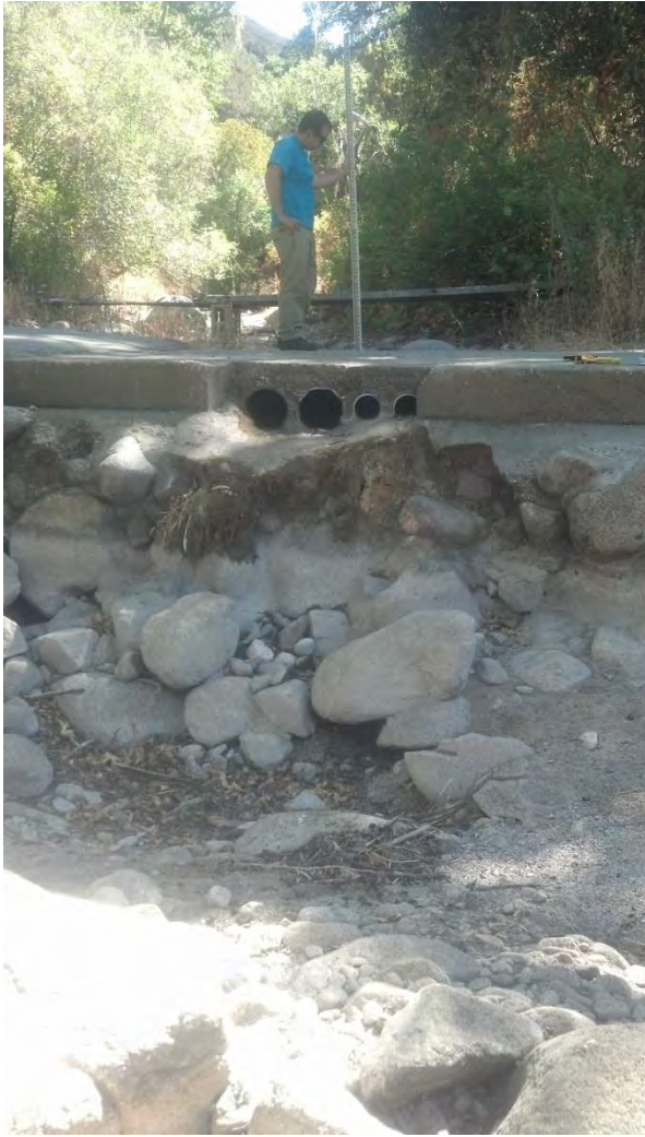
Site UCC-3. Left photo. Looking upstream at the culvert outlets and the ford drop-off. A seasonal plank walkway is shown in the background.
