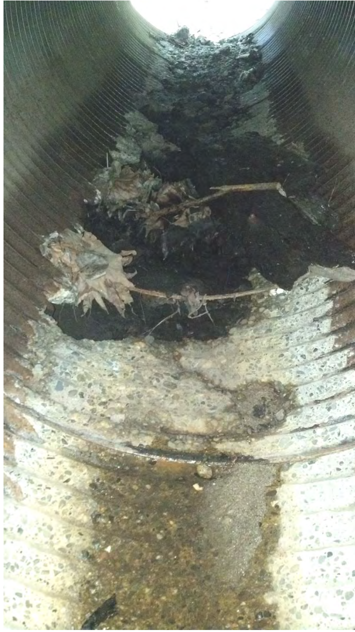
PCB-6. Interior of R/B culvert showing large section of rusted out pipe.
