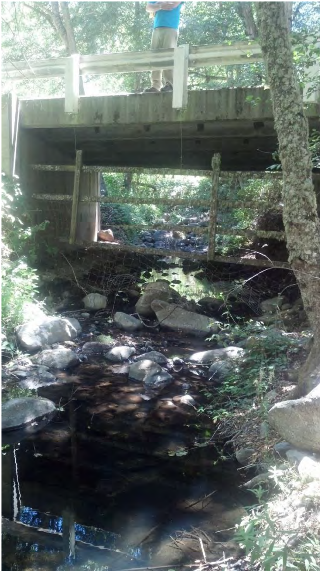
Site UCC-10. Looking upstream. Note the wood slat fence.
