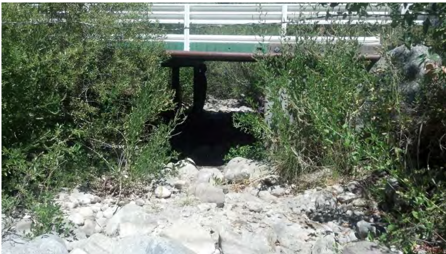
Site UCC-6. Looking downstream.
