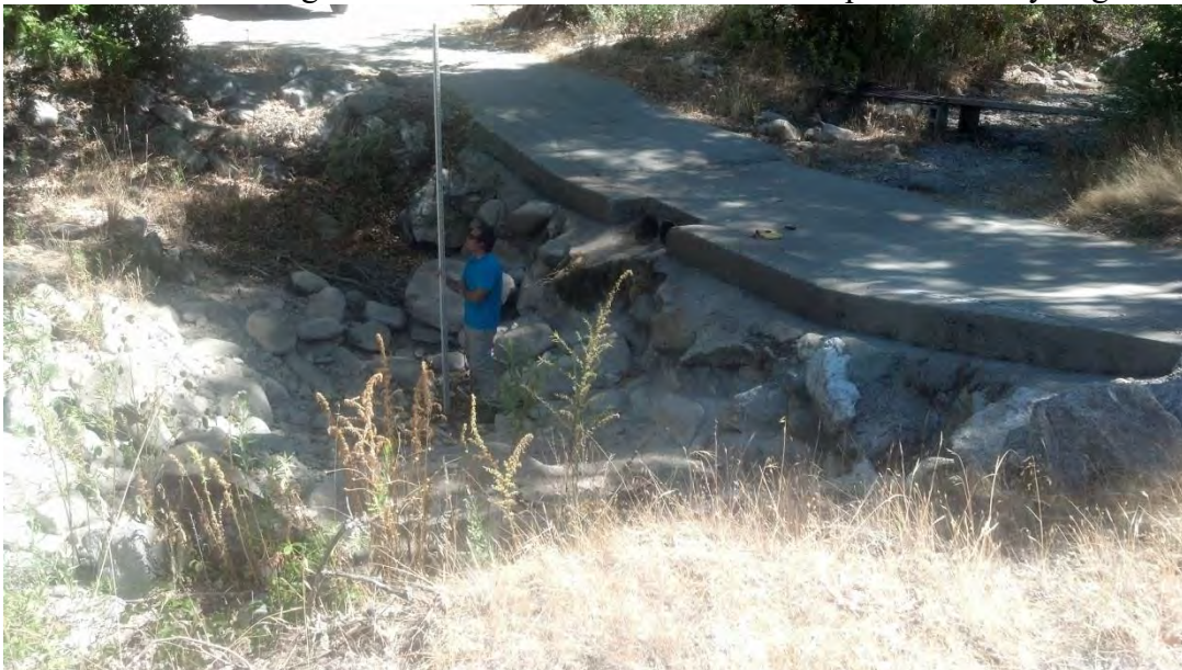
Site UCC-3. Looking across from l/b side.
