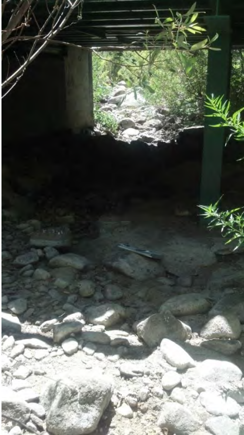
Site UCC-6. Looking upstream.
