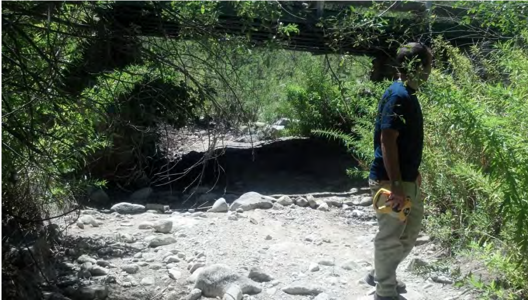
Site LCC-13. Looking upstream under bridge towards rock dam.
