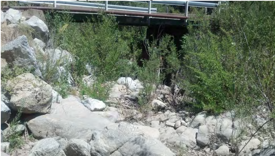
Site LCC-13. Looking downstream. Substrate is boulder/cobble, riparian vegetation is brushy.
