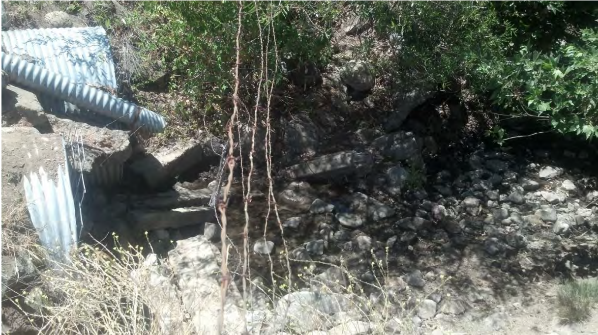
Site UCC-12. Looking downstream. Note concrete rubble at outlets.
