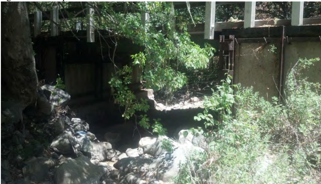
Site UCC-7. Looking downstream. Note the large sycamore tree on left side and boulder pile across the channel.
