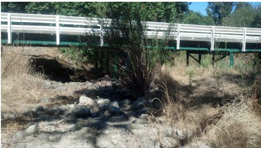
Site LCC-2. Nason Road Bridge. Looking d/s.
