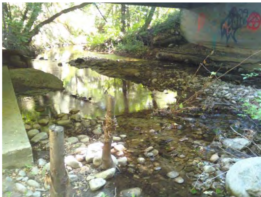
Site LCC-4. Shown at ~7 cfs. Split channel and sandbar under bridge. Looking upstream at abutments.
