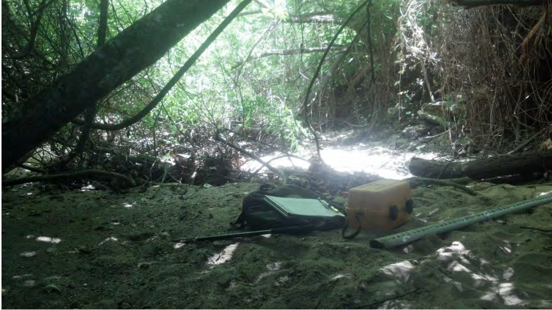
Site PCB-5. Plunge pool and d/s channel from culvert outlet.
