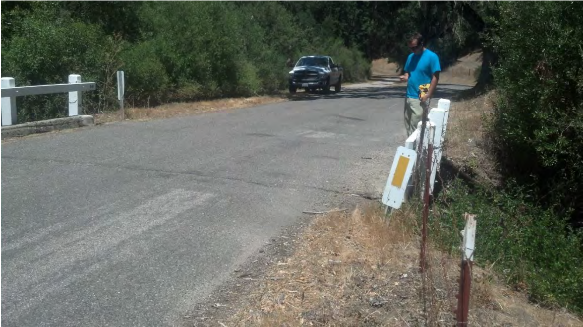
Site UCC-11. Small MoCo. Bridge.
