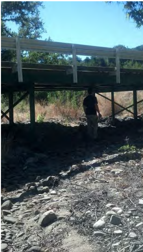
Site LCC-2. Nason Road Bridge. Looking u/s.
