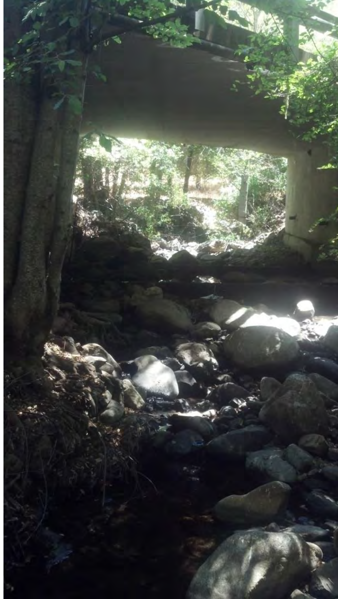
Site UCC-8. Looking upstream.
