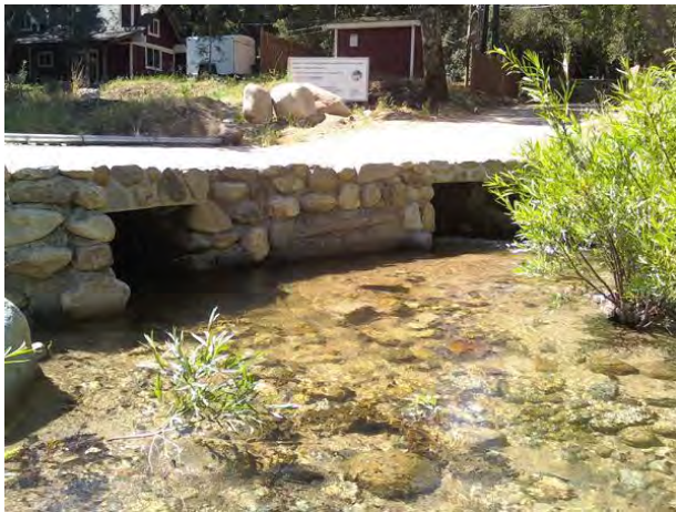
Site LCC-3. Outlets.
