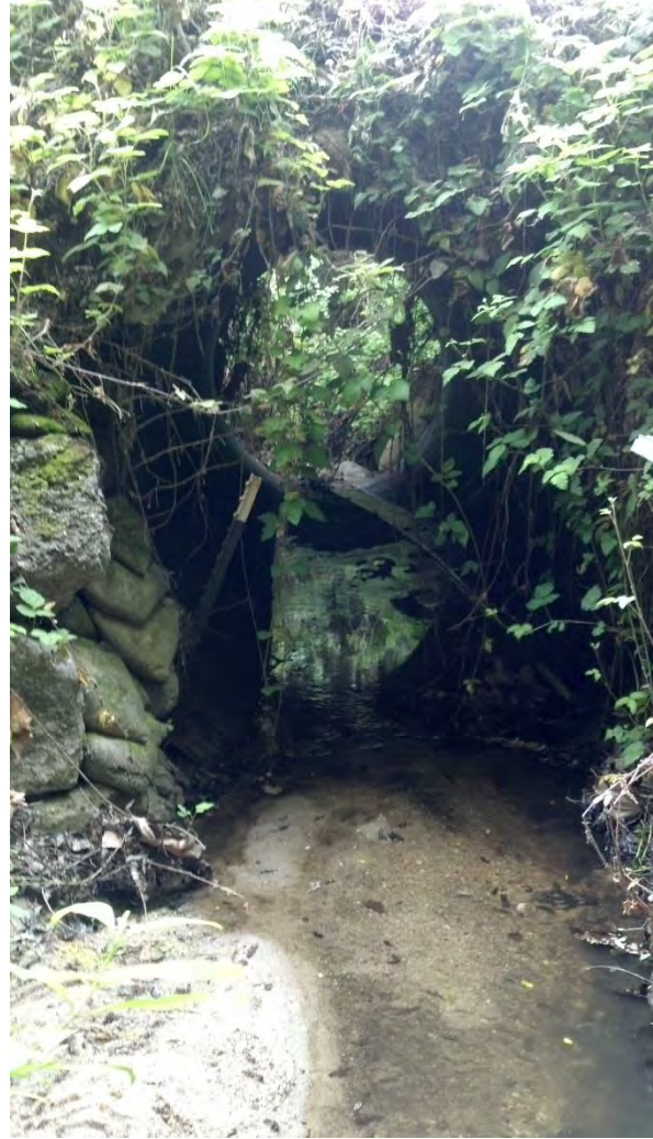
Site PCB-7. Photo #3. Looking d/s through culvert. Photo #4. Culvert inlet showing the narrow concrete and T-post entrance and sandy substrate.
