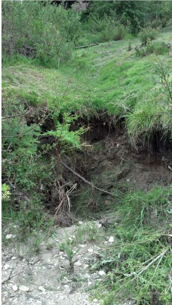
Site PCB-2c. Deep scour hole above rock weirs.
