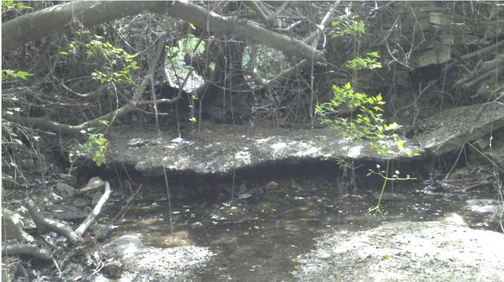
PCB-6. Outlet apron and drop off.
