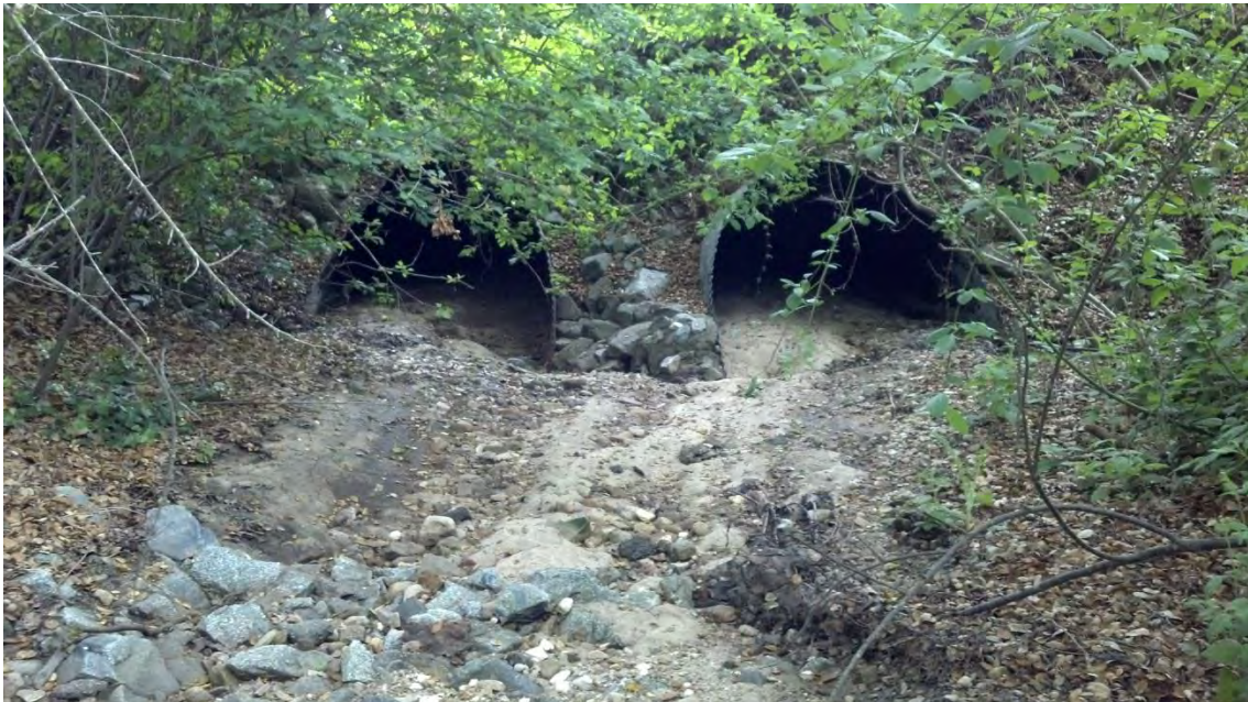
Site PCB-3. Valley Greens Rd. culverts - Looking downstream.
