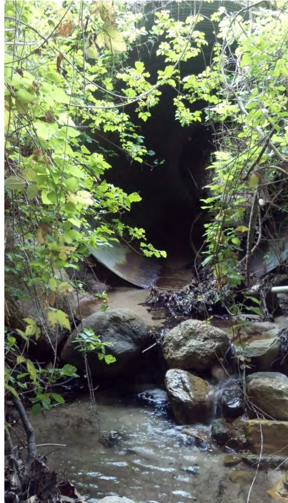
Site PCB-7. Photo #1. Looking d/s at brush and sandy substrate below the culvert. Photo #2. Culvert outlet showing the boulder weir and sand apron.
