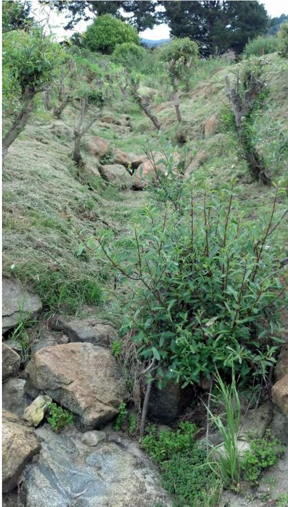
Site PCB-2c. Steep rock weirs
