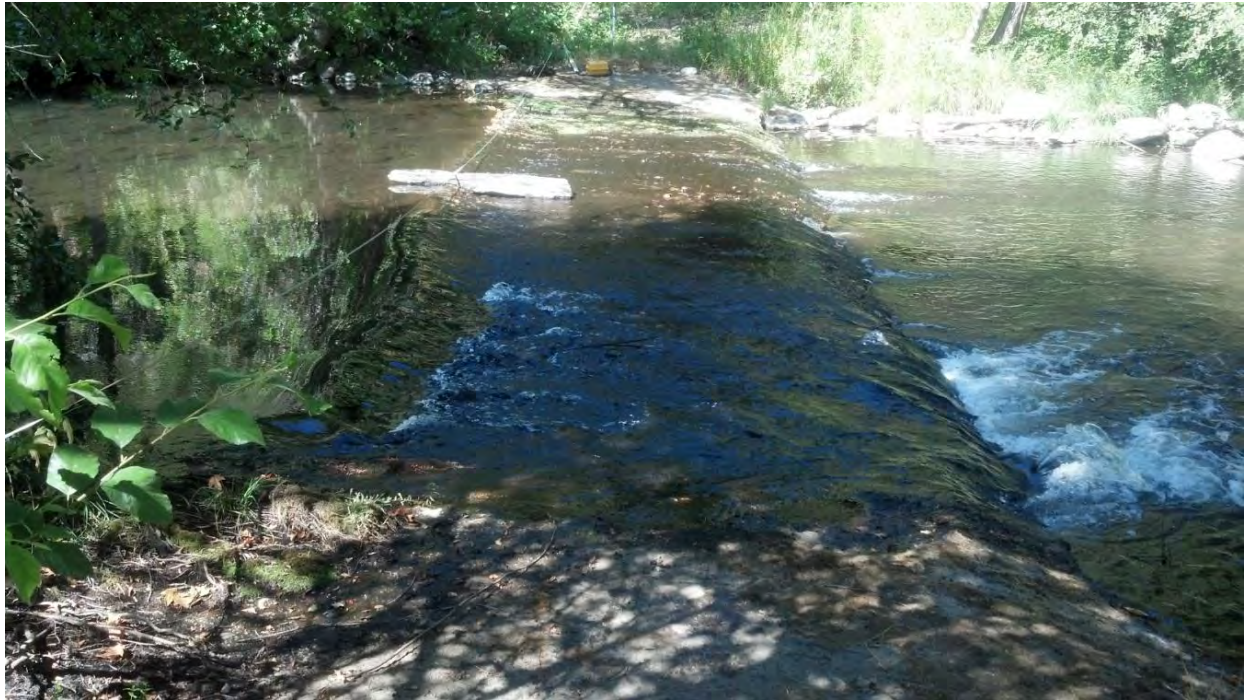
Photo 1) Looking across the ford from right bank. Note the exposed rebar along upper/rightbank side of ford (white water area in foreground).
