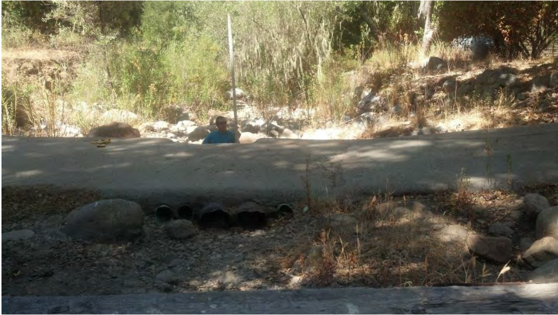
Site UCC-3. Looking downstream at the culverts and plunge pool drop-off.
