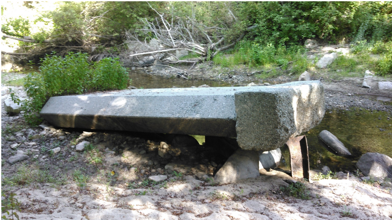
Concrete bridge pier to be removed
