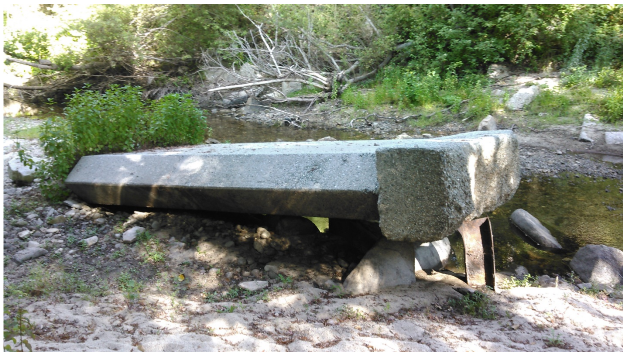
Concrete bridge pier to be removed
