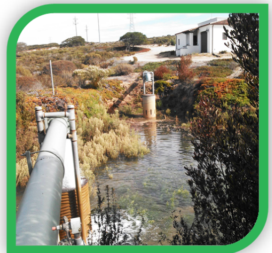
Above - New Monterey Pipeline under construction to facilitate distribution of water from the Pure Water Monterey project, and transmit excess Carmel River water to ASR wells in the winter. Below – Backflush pit at ASR site. 699 AF of Carmel River water were injected for storage in the Seaside Basin in 2016.
