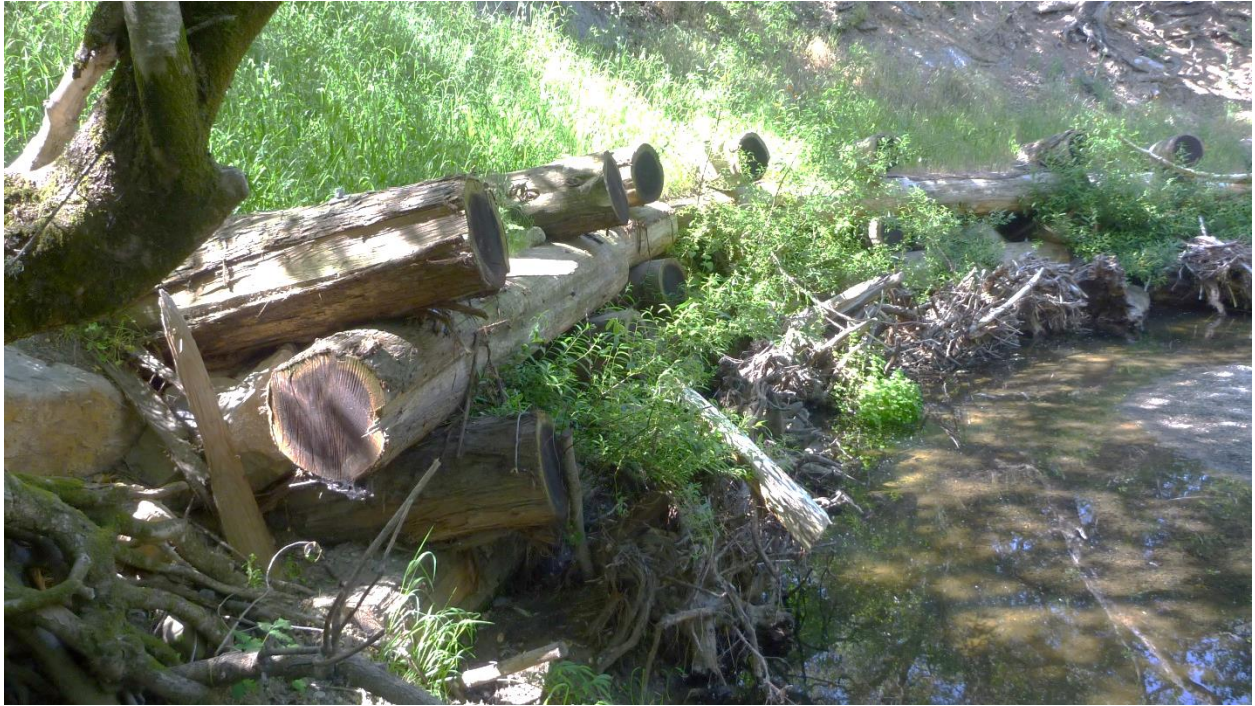
Figure 6. Example of completed log crib wall
