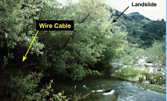
As streamside plants mature, the post and wire is incorporated into the trees and can provide significant protection; however, after several years, the posts rot at the toe of the slope. This reduces the effectiveness against erosion and can be a liability if the wire mesh and posts move downstream and clog the channel. In addition, fisheries biologists object to wire mesh placed near the path of migrating adult steelhead.
