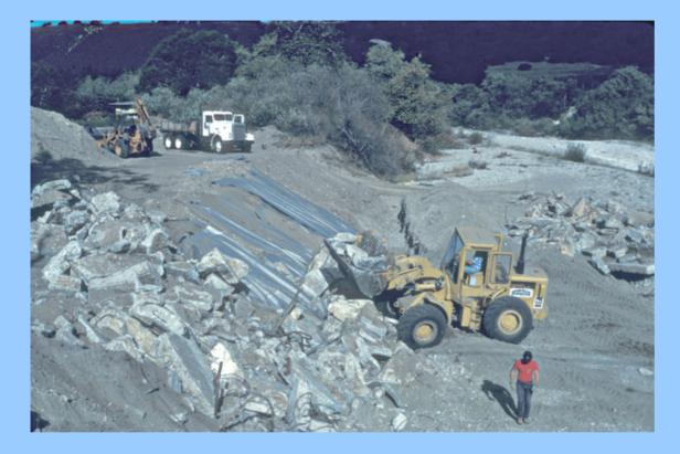
Right – a close up near the loader bucket, showing what appears to be green sticks amongst the rubble. Willow cuttings were integrated into the slope protection from the beginning. Restoration work was carried out in three phases, with work at the bridge scheduled first. Here, concrete rubble is placed on a streambank rebuilt with native river material. The shiny black cloth under the rubble is used to stop fine strambank material from washing out during high flows.
