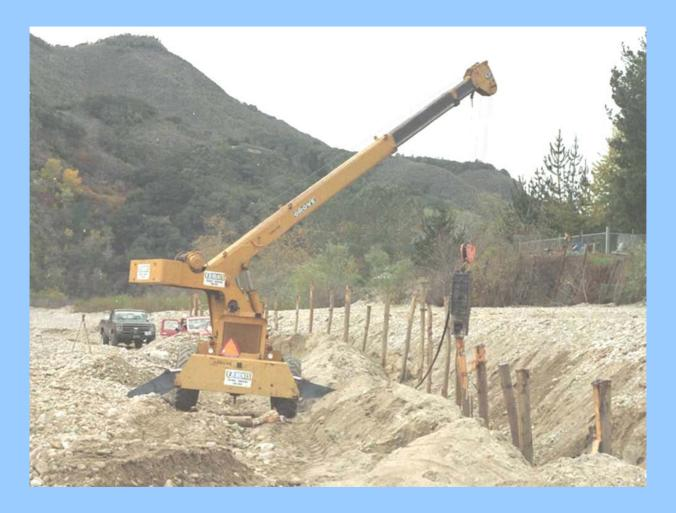
Above - 12-foot long eucalyptus posts were sunk at 10-foot centers at the toe of the streambank along the outside of bends. This provided the framework to place six-foot wire mesh that resembled chain link fence. About three feet of the mesh was buried below the streambed to resist toe scour. This method worked fairly well at the Schulte Project, as a drought between 1987 and 1991 allowed vegetation to become established enough to resist high flows.
