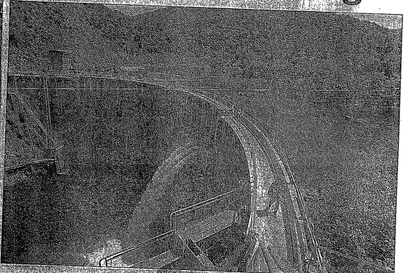
Water is released through a series of holes that were drilled into San Clemente Dam in Carmel Valley. Cal Am officials estimate the dam may be in danger of collapsing if a large earthquake occurred. Fred Faizollahi, senior operations engineer, walks across the San Clemente Dam. VERN FISHER/Herald File
