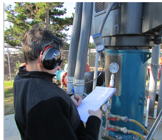
Joe Oliver, MPWMD Water Resources Manager collection data at ASR Well # 3. Enough water to serve 1,450 homes for a year has been stored for later use by the ASR project.
