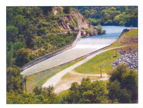
Water Project #5 explores the possibility of expanding capacity of the Los Padres Reservoir via dredging and/or a small increase in spillway elevation. The increase in spillway elevation could perhaps be achieved by a rubber dam.
