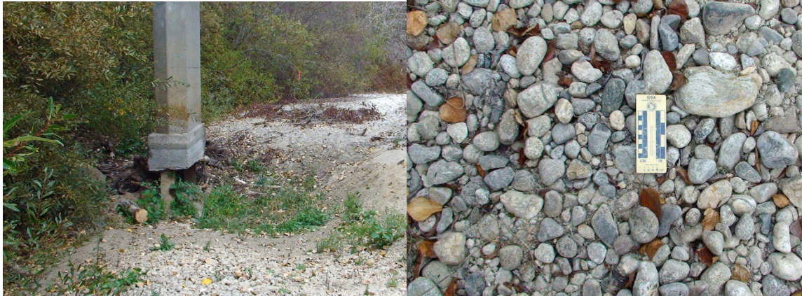
Bridge pier at Rancho Canada Golf Course Cart Path (~RM 2.7) showing scour and typical gravel bed material (photo by R. Mussetter, November 7, 2007). Contrast with sand/fine gravel gradation from 2001 samples in Figure 1.
