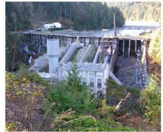
Elwha Dam Port Angeles, WA
