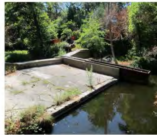
Lagunita Dam Palo Alto, CA
