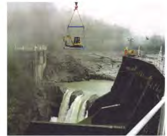
Glines Canyon Dam Port Angeles, WA
