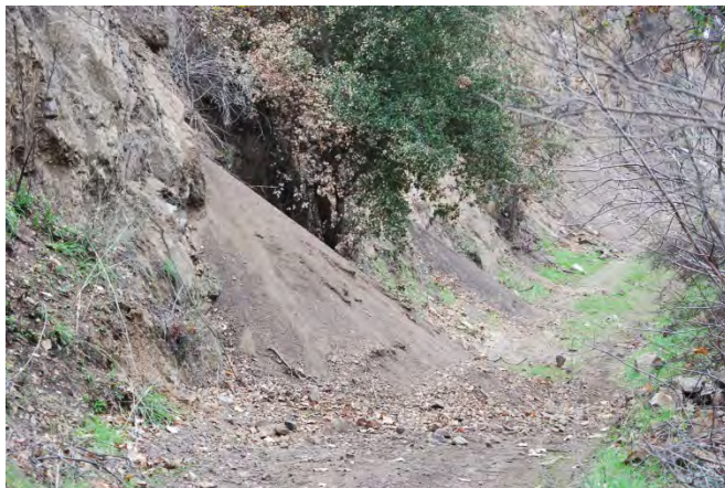
Sediment sluffing off slope at LPD following 2016 Soberanes Fire
