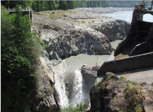
Glines Canyon dam removal
