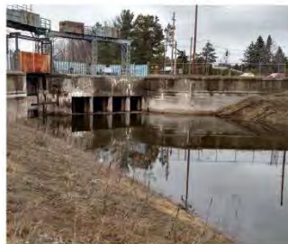
Boardman River Dam Traverse County, Michigan
