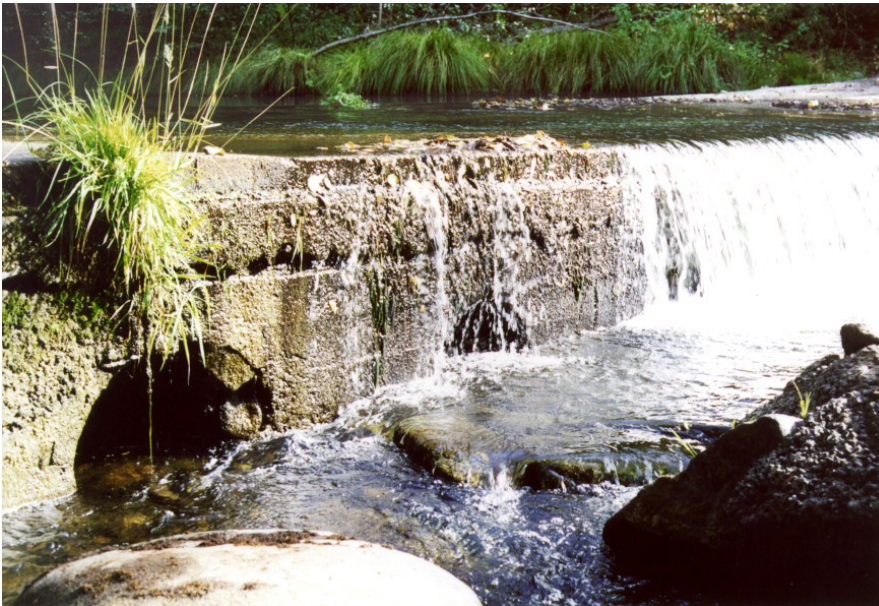
Looking upstream from north side (above)
