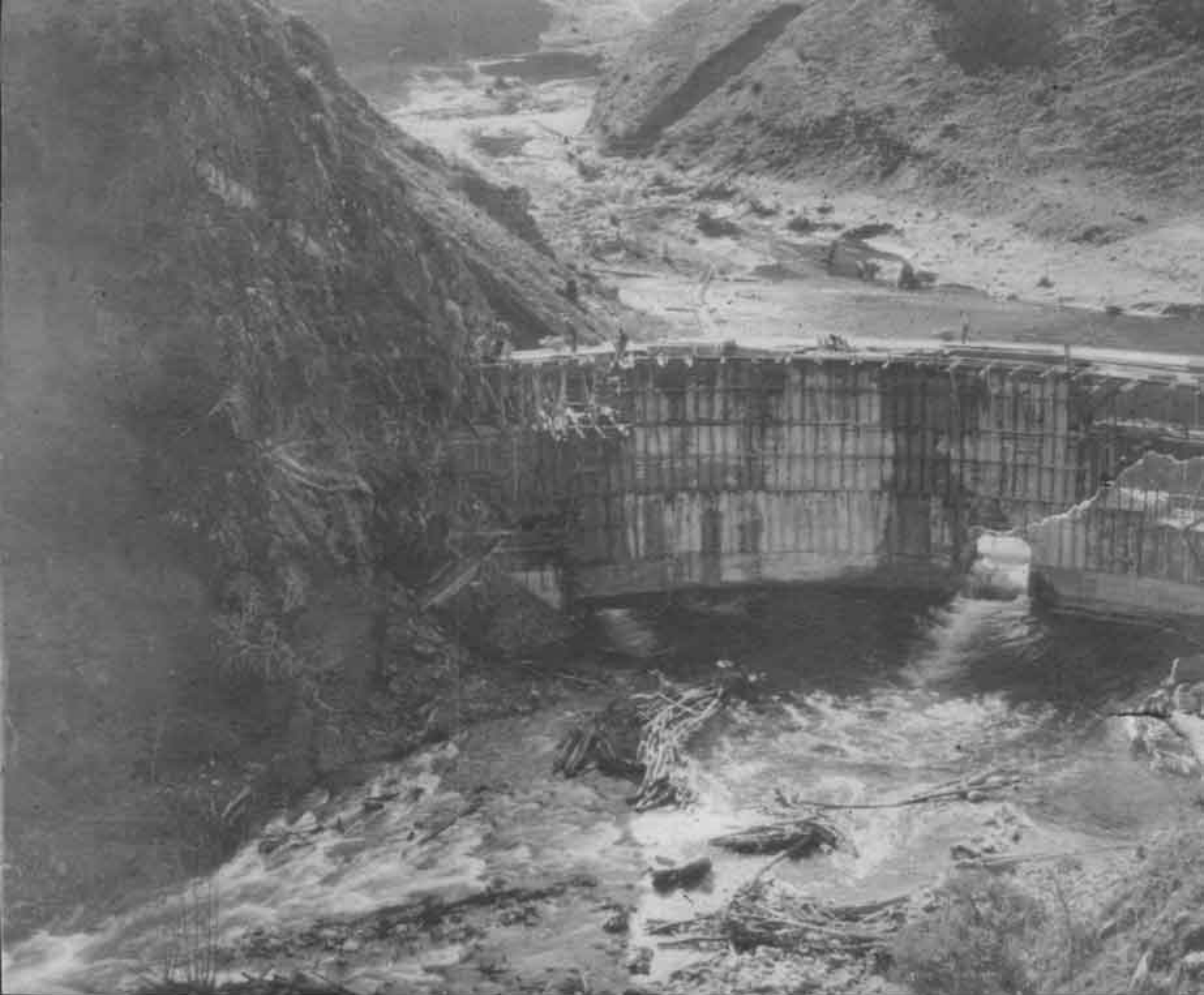
San Clemente Dam under construction in 1921.
