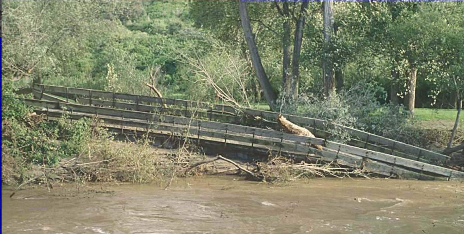
Rancho Cañada Bridge No. 5 1994 (left) 1995 (below)
