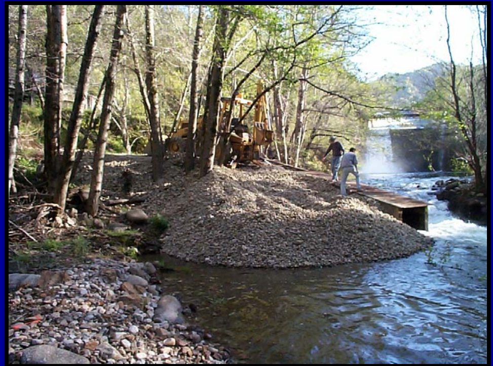
A backhoe pushes spawning gravel into pool near fish ladder.
