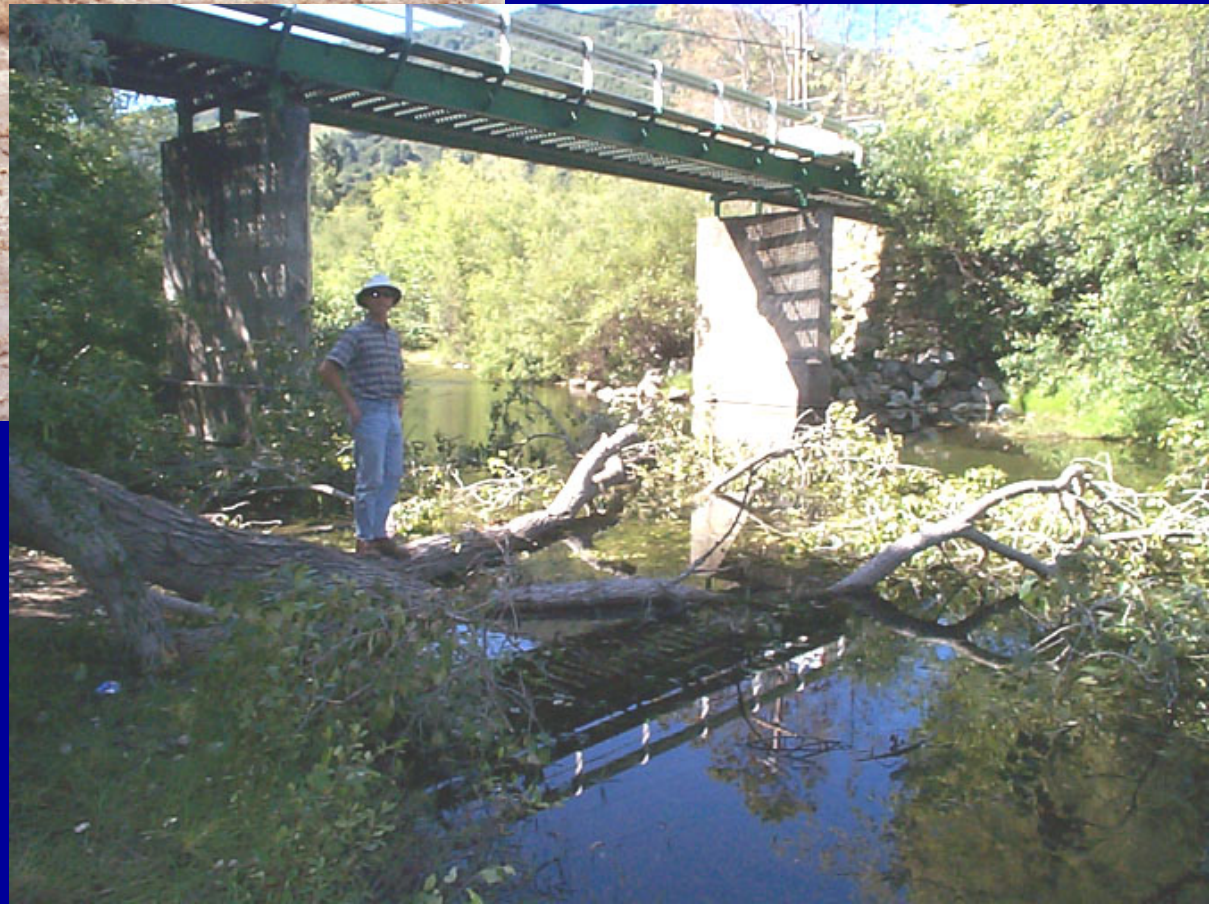
MAY 2002 BORONDA BRIDGE (right)
