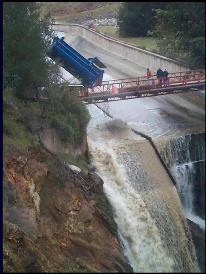
Placing spawning gravel through the bridge at the Los Padres Dam spillway.
