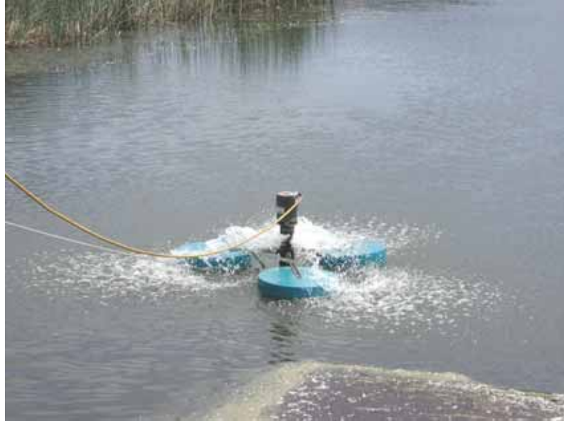
Figure 10.13 The first of two aeration machines installed in the South Arm of the Carmel Lagoon during the fall. Photo: Joel Casagrande, 01 Sep 03
