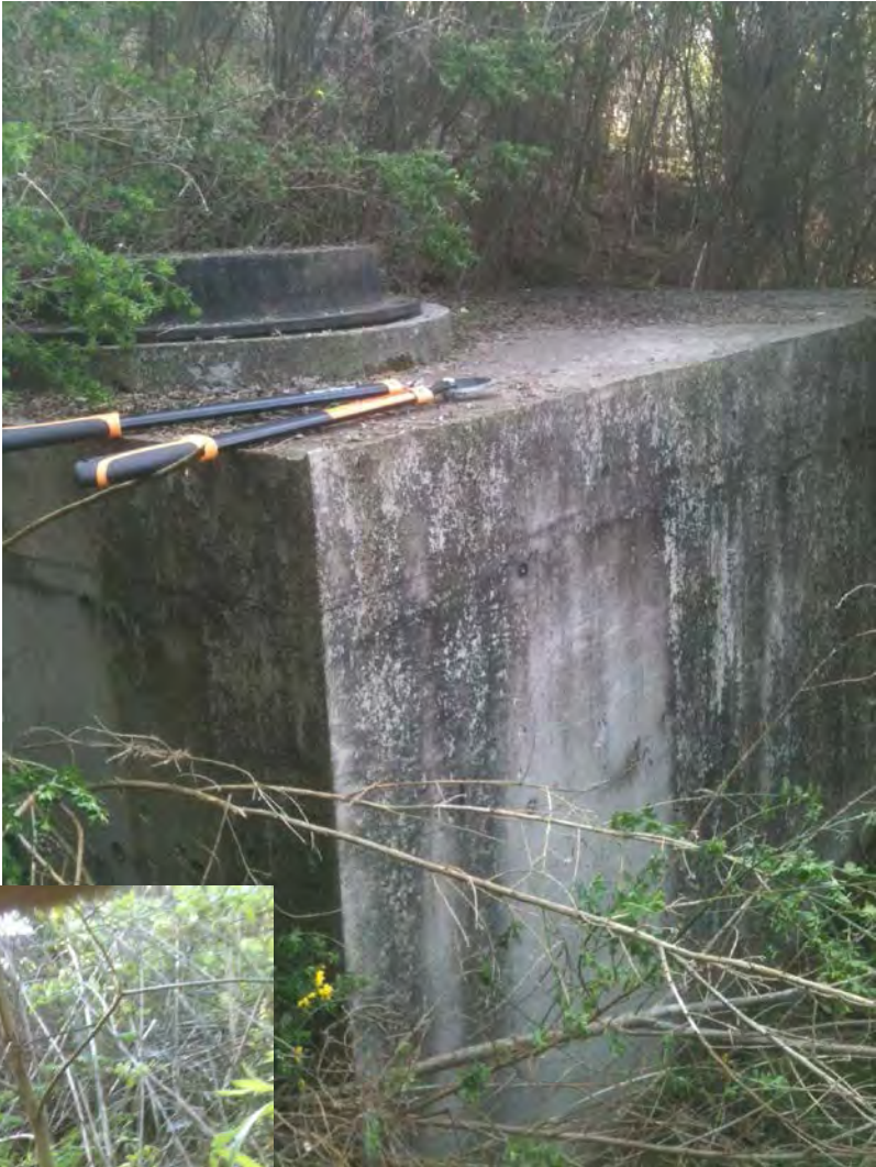
09_C_01 – Outlet Structure and Manhole
