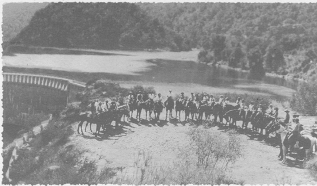
San Clemente Dam • March 29, 1932
