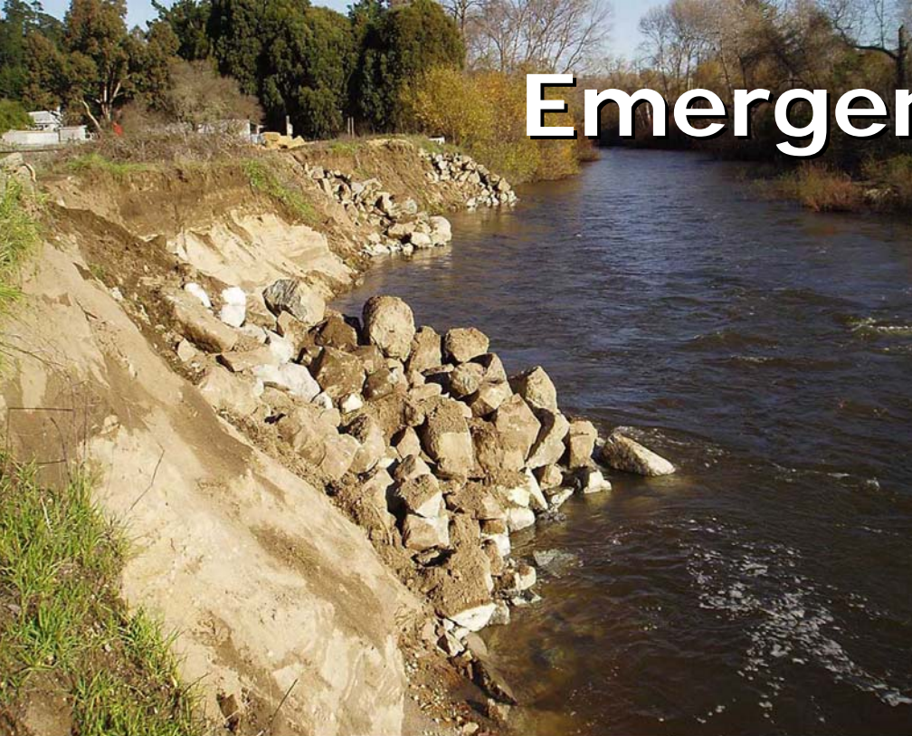
Above - after rock placmeent on January 13, 2005. Below - during erosion on January 9, 2005
