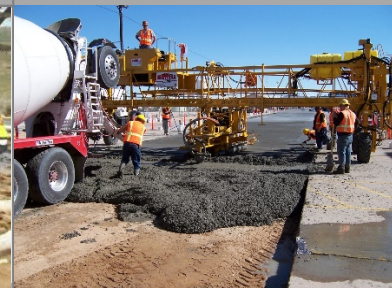
Earthwork, Concrete & Asphalt Paving
