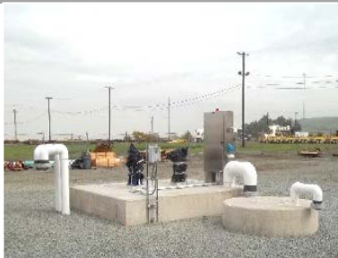
DB Replace Sewer Lift Stations
