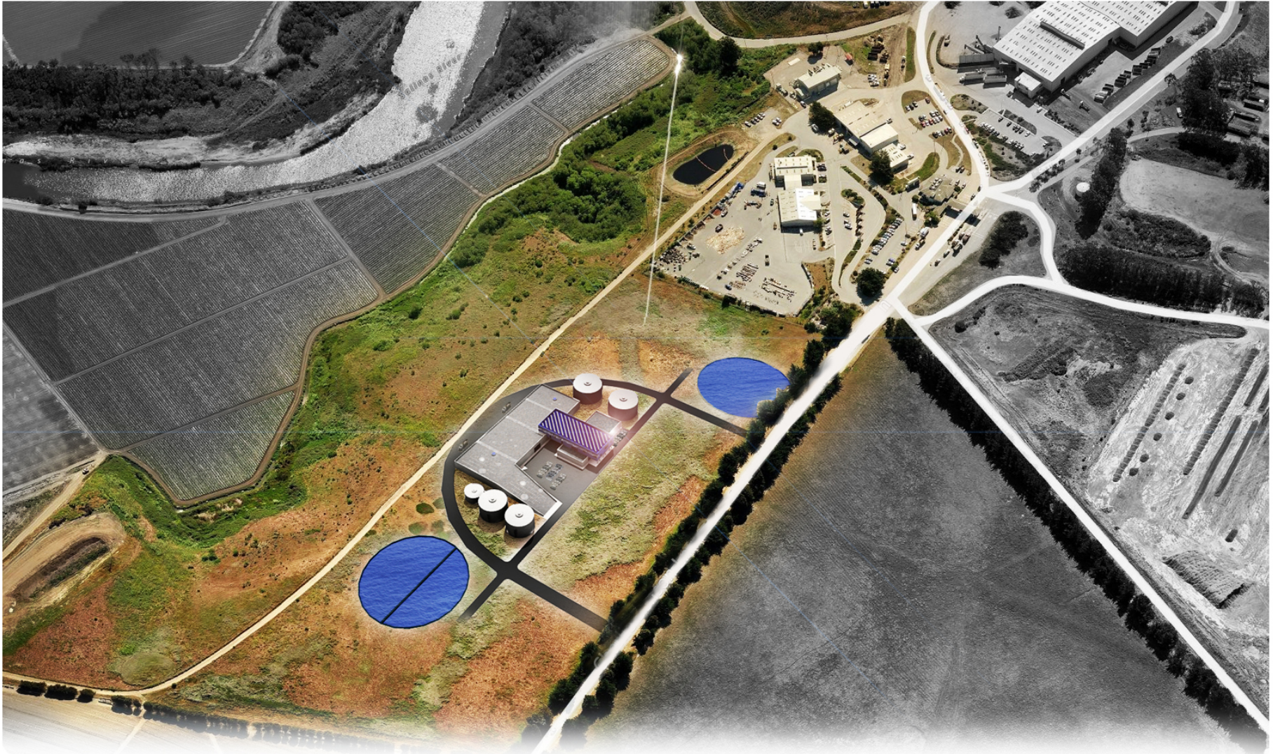
MPWSP Desalination Plant
