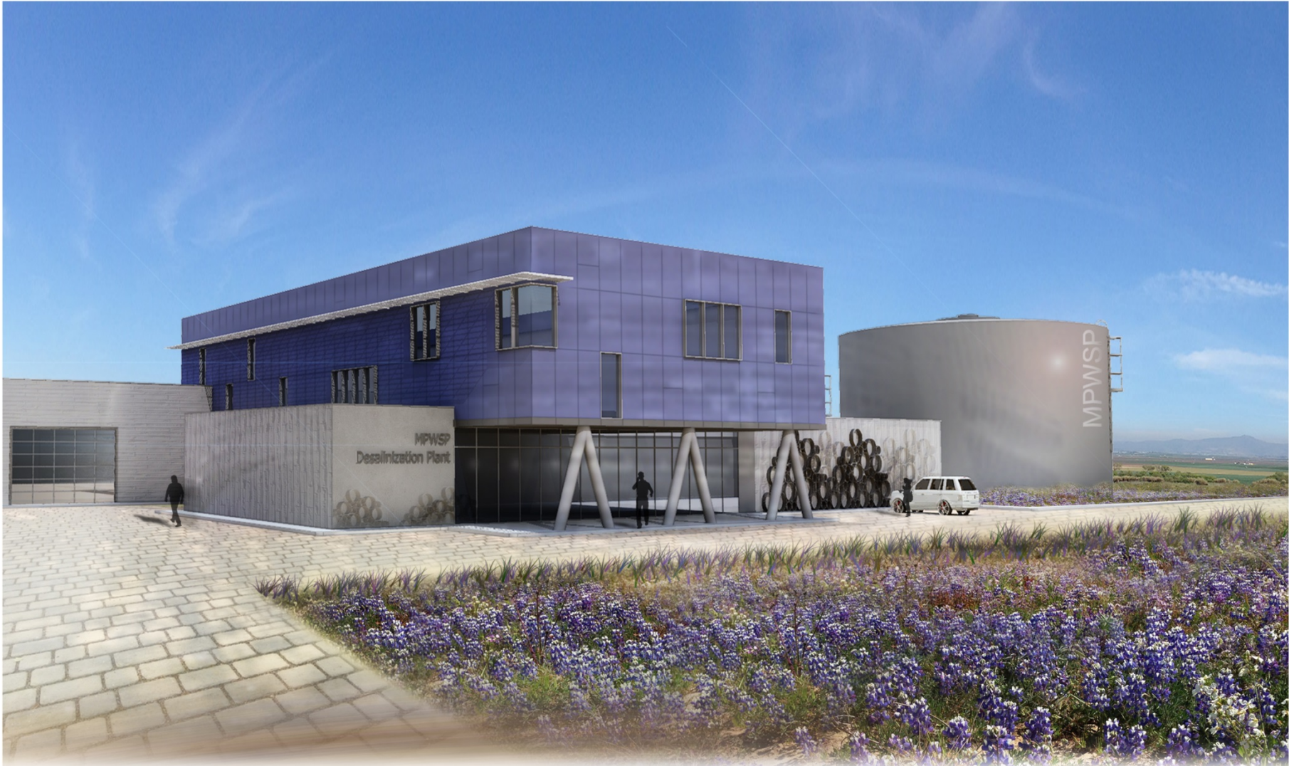
MPWSP Desalination Plant
