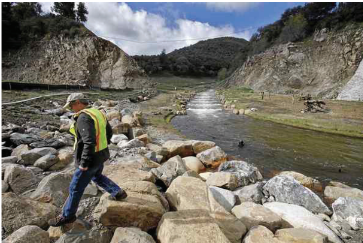
NOAA research ecologist Dr. David Boughton walks along the new Carmel River channel with step pools and resting pool at the former San Clemente Dam site on Thursday. (Vern Fisher - Monterey Herald)
